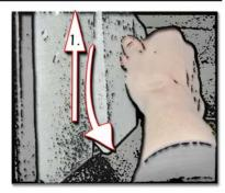
3. Lift the stone upwards about 5 to 7 mm by means of the screwdriver. Then let the stone somewhat down and twist the lower part inwards towards the fireplace and then let it down entirely.
